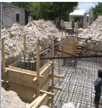
Torre Telcel Sierra P.
